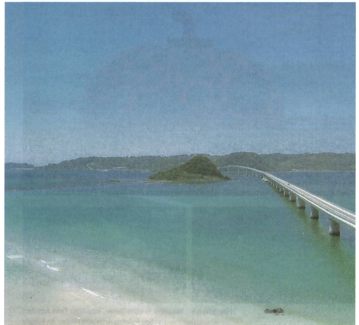
Tsunoshima Ohashi Bridge
