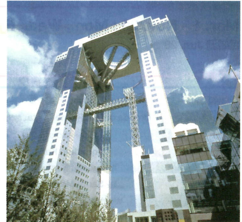
Aerial Garden Observatory
